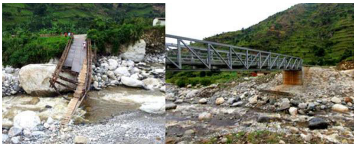
Bridge at Nyamwamba project site reconstructed (right) after the severe flood damages in 2014 (left).
