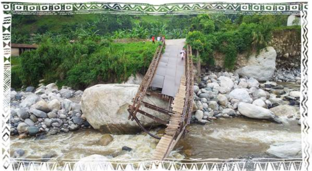
Flood damages at Nyamwamba documented during GET FiT Supervision visit in June 2014 (Photo: GET FiT)
